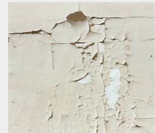
Loose and cracked plaster left, skim coat peeling right
