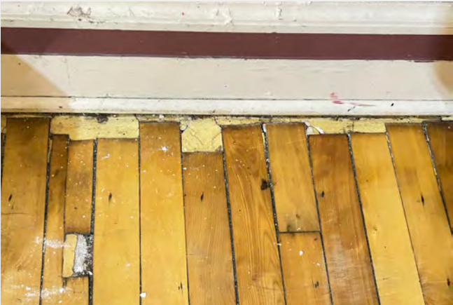
House main level wood floor ‘fillers’
