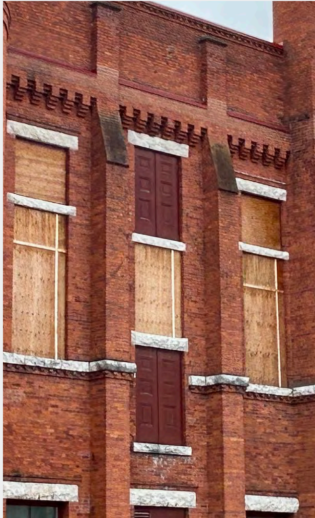
Efflorescence and staining on brick masonry
