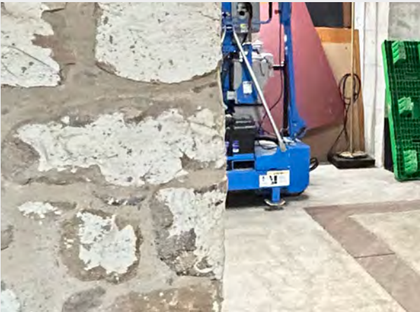
Stone masonry foundations
