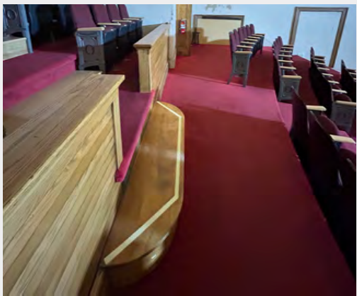
Wood step and guard house balcony level, with refinishing and visibility strip on right.
