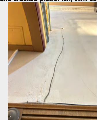
Exposed electrical wiring
