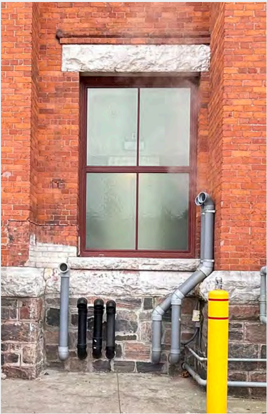
Main level two over two windows
