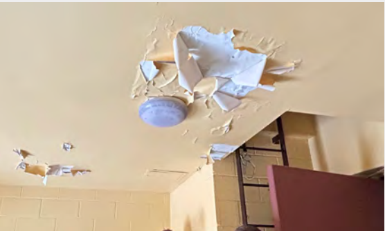
House Exit Stair damaged plaster ceiling.
