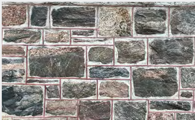
Ribbed joints at stone masonry foundation
