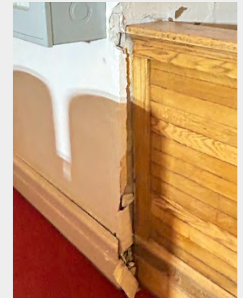
Loose and cracked plaster at balcony wall and guard
