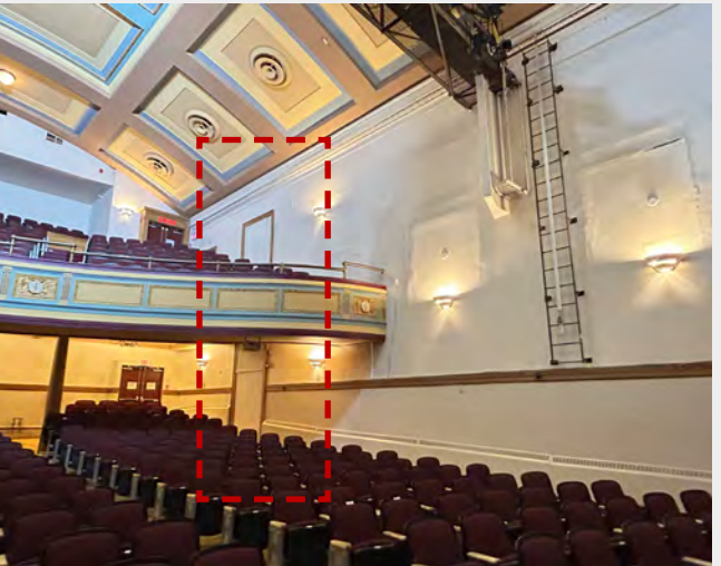
Former fire escape access (inside dashed lines) and telescoping plaster at previous windows to the right.
