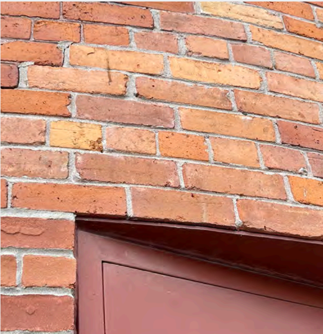
North elevation bricks showing holes, cracks and incompatible mortars.
