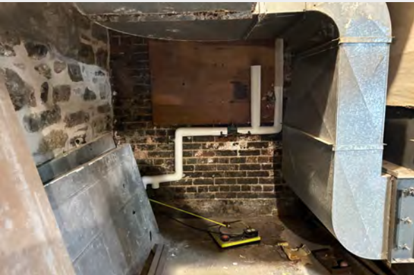
Fan Room, brick walls with efflorescence
