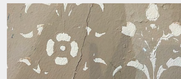
Foyer Stairwell paint stencil deterioration.
